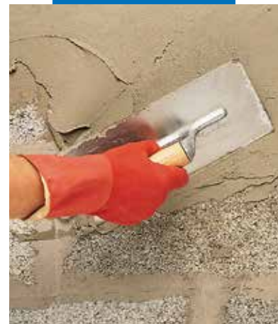
Nanošenje Planiseal 88 gletericom
